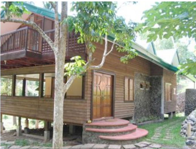
Above: One of the new buildings
