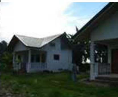
New houses for children – almost finished
