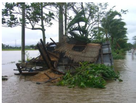
Above— house destroyed by storm
